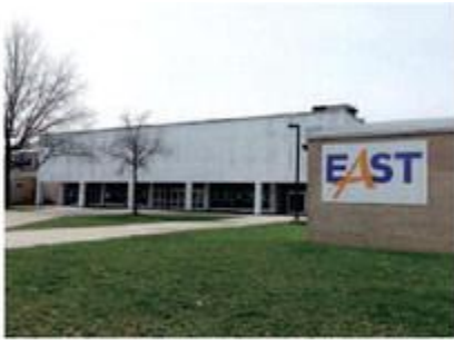
An exterior of East High School. JAMIE GERMANO/@JGERMANO1/STAFF PHOTOGRAPHER
